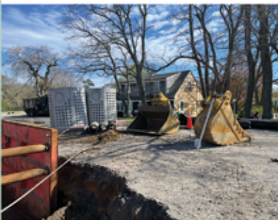
Two leech pits solve the parking lot flooding.
