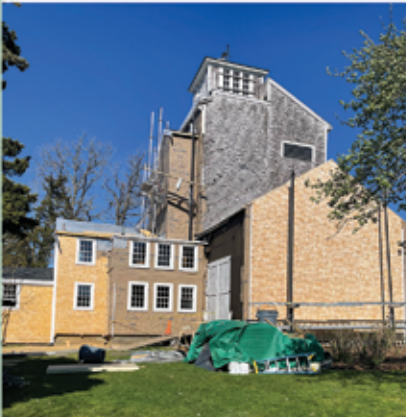
New insulation & cedar shakes preserve the Playhouse.
