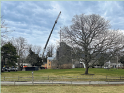
A crane lowers the first steel column through the roof.
